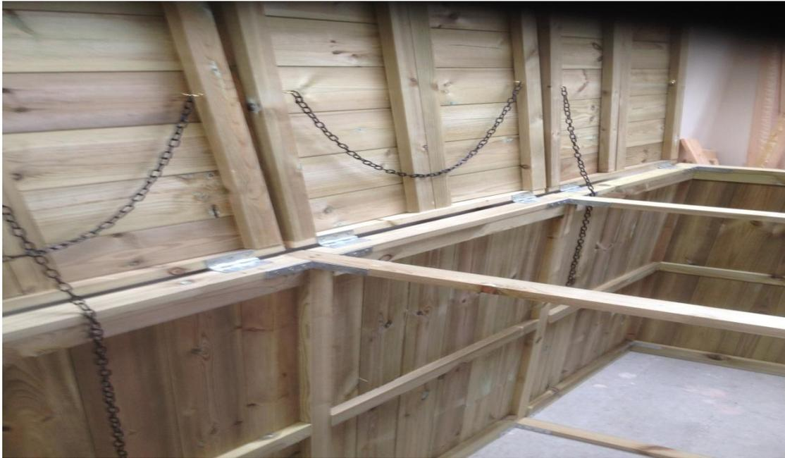
**Step 6:** Take the right hand panel marked 6 and slot into the back panel also marked 6, Fix using 2 metal brackets, one near the top and one near the bottom, with the 1" brass screws until the two panels are tight.
