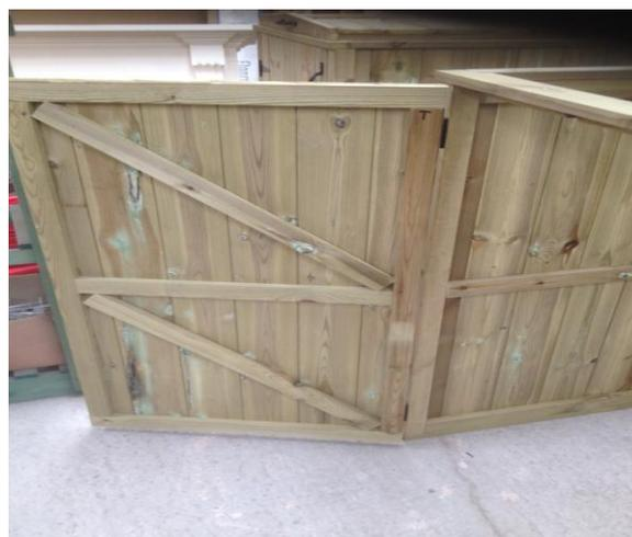
**Tip D-** When fitting the hinge to the door, use the smallest screw provided in the end hole of the narrowest part of the hinge.
