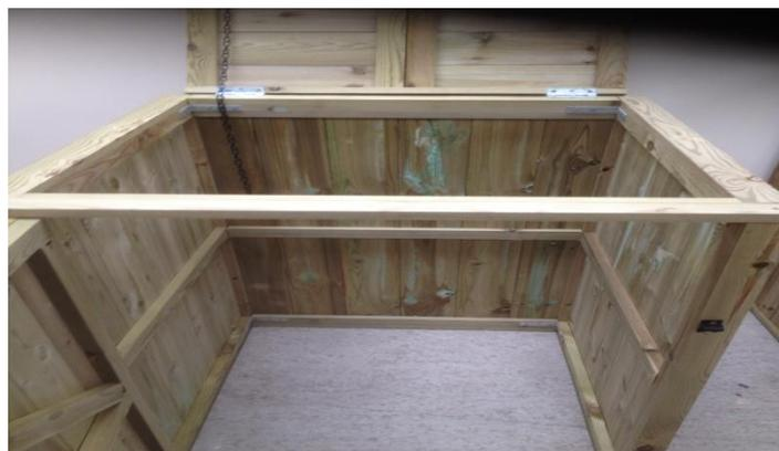
**Step 3:** Lay the front bar in position across the front of the screen, match A to A and B to B with the overhang to the front. Fix from the top using 2 brass screws, 1 at either side using the pre-drilled holes.
